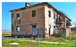
Image A.2-1: Housing situation on Pirallahi Island 19
