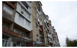
Image A.3-1: Typical multi-story building in Nefchala without access to water during drought (source: Anar Vallyev)
