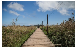
Image I.2-4. Wooden Bridge in Bandar Kiasahr
