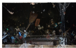
Image A.2-4: Basements of some residential buildings in Pirallahi district are flooded 22
