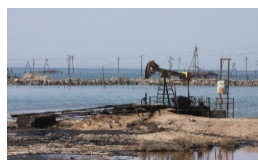
Image A.2-3: The site has been area of extensive oil exploitation and left with many dilapidated equipment 21
