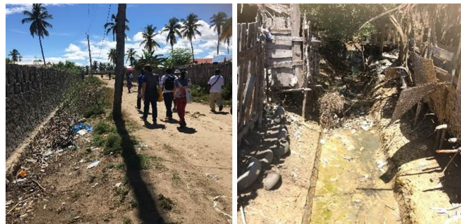
Figure 10: Drainage conditions in Morondava
