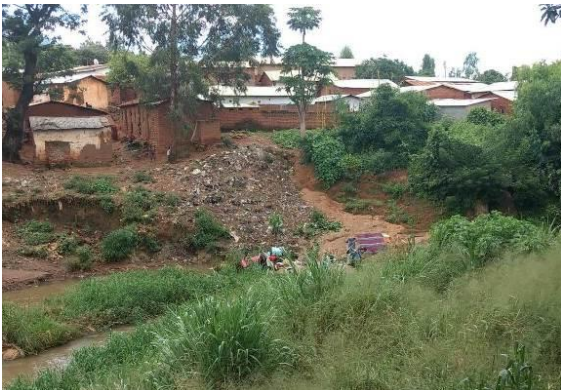
Figure 16: Encroachment of settlements near the Likangala River
