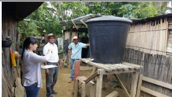
Rainwater collection system, Las Chispas Township.
