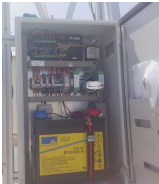
Figure 9: Control box with datalogger, battery and electric equipment
