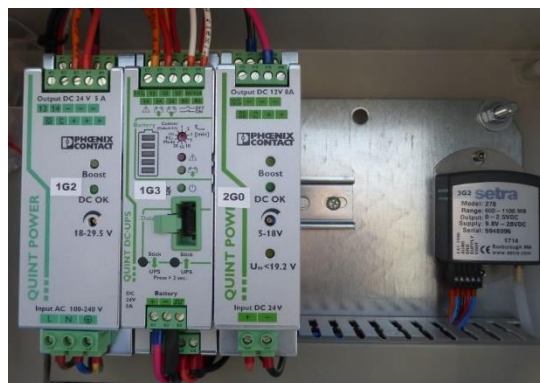
Figure 8: UPS and Setra 278 pressure sensor
