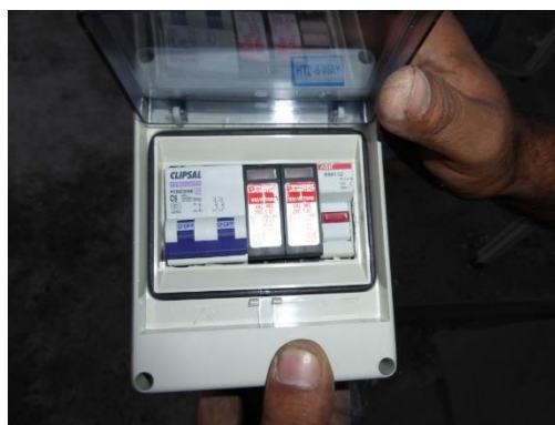
Figure 12: Circuit breaker and power surge protection
