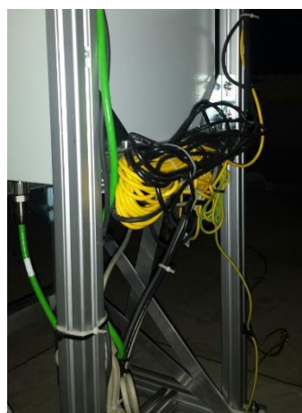
Figure 14: Excess cable storage on control box
