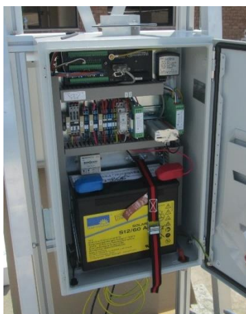
Figure 9: Control box with datalogger, battery and electric equipment
