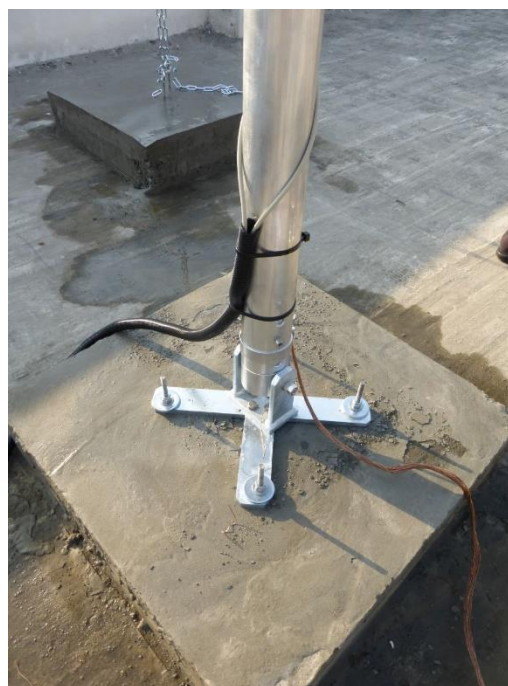
Figure 14: Wind tower base
