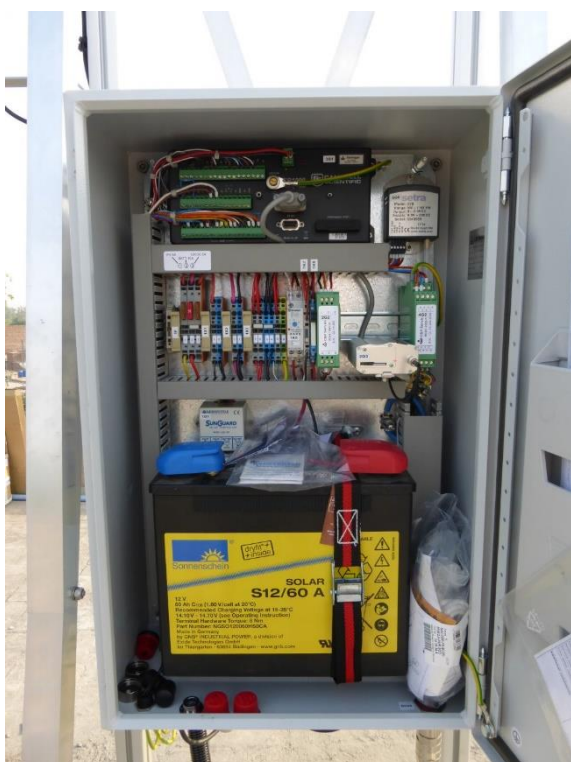
Figure 9: Control box with datalogger, battery and electric equipment
