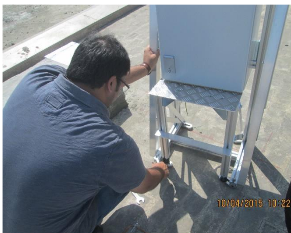
Figure 5: Installation of support structure
