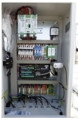
Figure 9: Control box with datalogger, UPS and electric equipment
