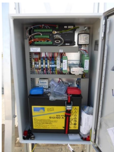
Figure 5: Control box with datalogger, battery and electric equipment
