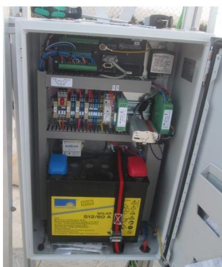
Figure 9: Control box with datalogger, battery and electric equipment
