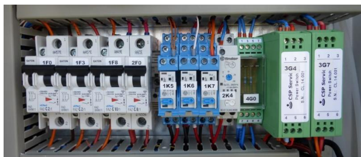
Figure 12: Circuit breakers and automatic switches
