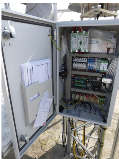
Figure 9: Control box with datalogger, UPS and electric equipment
