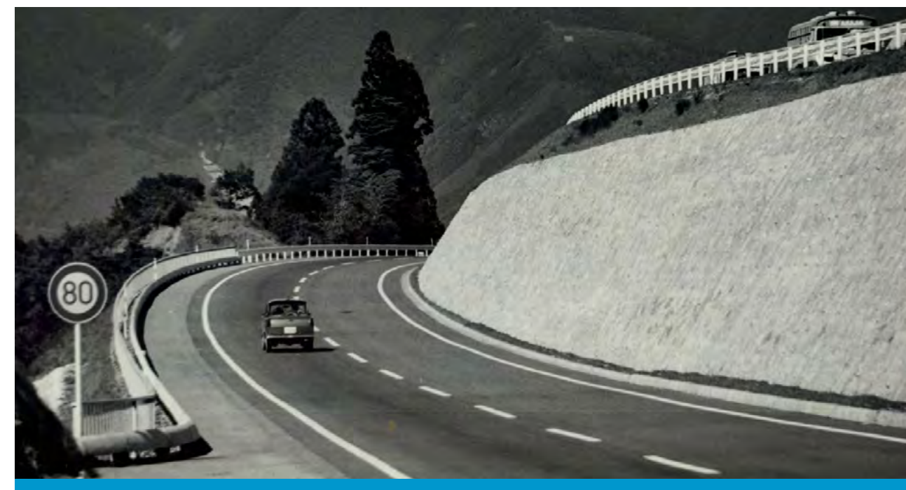
A view of the expressway between Kyoto and Hikono, part of the Tokyo-Kobe Expressway. The World Bank made several loans to the Nihon Doro Kodan (Japan Highway Public Corporation) to help finance the construction of the 335-mile toll express highway between Tokyo and Kobe. Photo © United Nations / World Bank Archives
