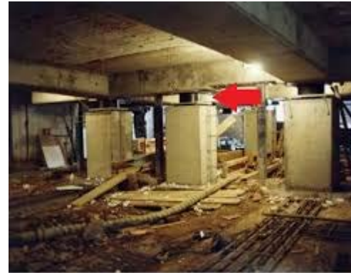
Strengthened foundation with base isolators inserted
