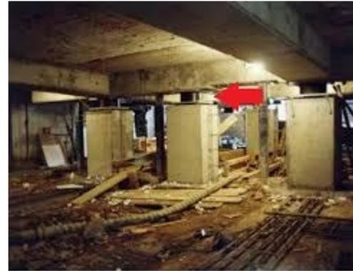
Strengthened foundation with base isolators inserted
