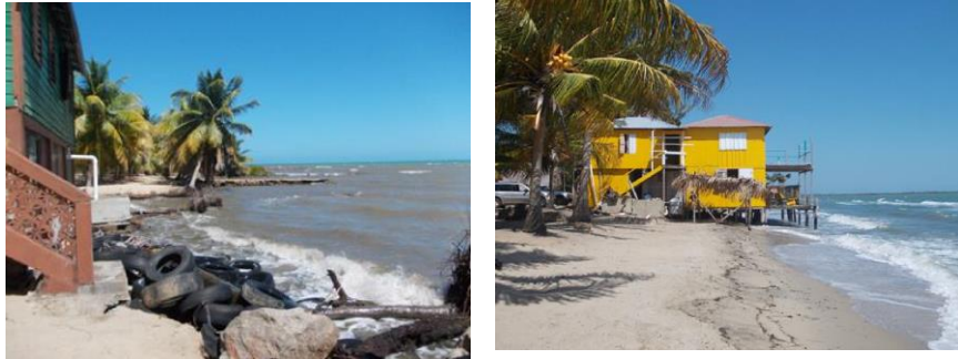
Figure 7: Images depicting erosion in Dangriga and Hopkins, respectively (NCCO, 2019)
