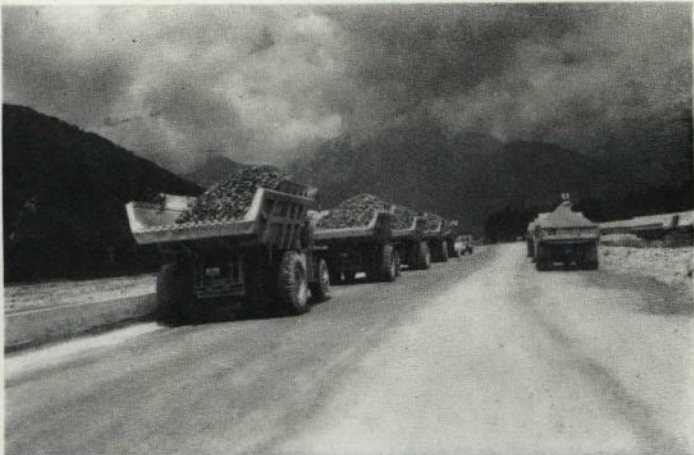
Kurobe. No. 4 Dam project : Aggregate transportation route
