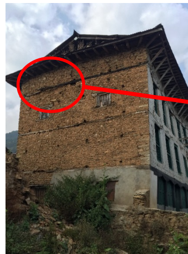
Houses with seismic band has less failure
