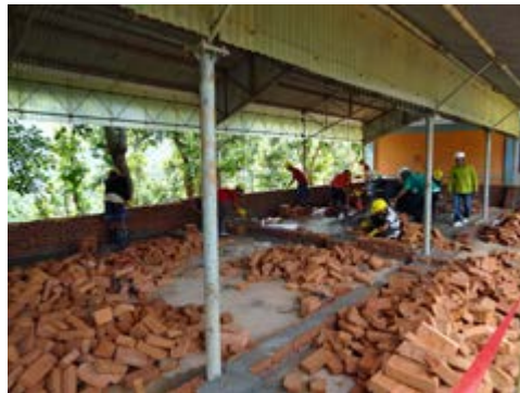
Repairs progress at a rapid pace.
