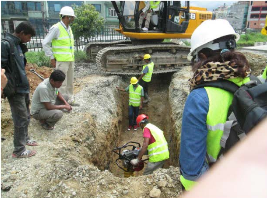
Eastbound Lane Back-filling and Compaction for an Open Crack July 20, 2015
